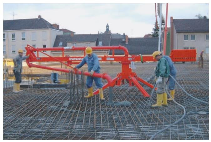
Mechanical distributors lend themselves perfectly where placement using truck-mounted pumps and stationary placement booms reach their technical and costefficient limits; i.e.
